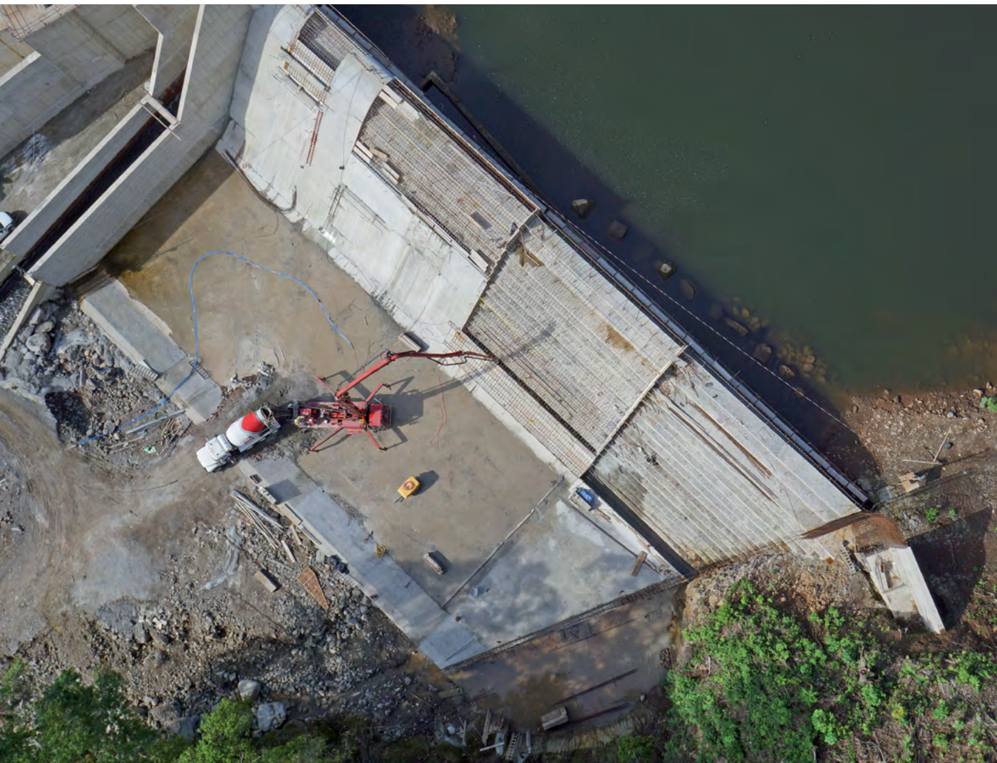
Costa Rica - Los Negros II hydroelectric plant
