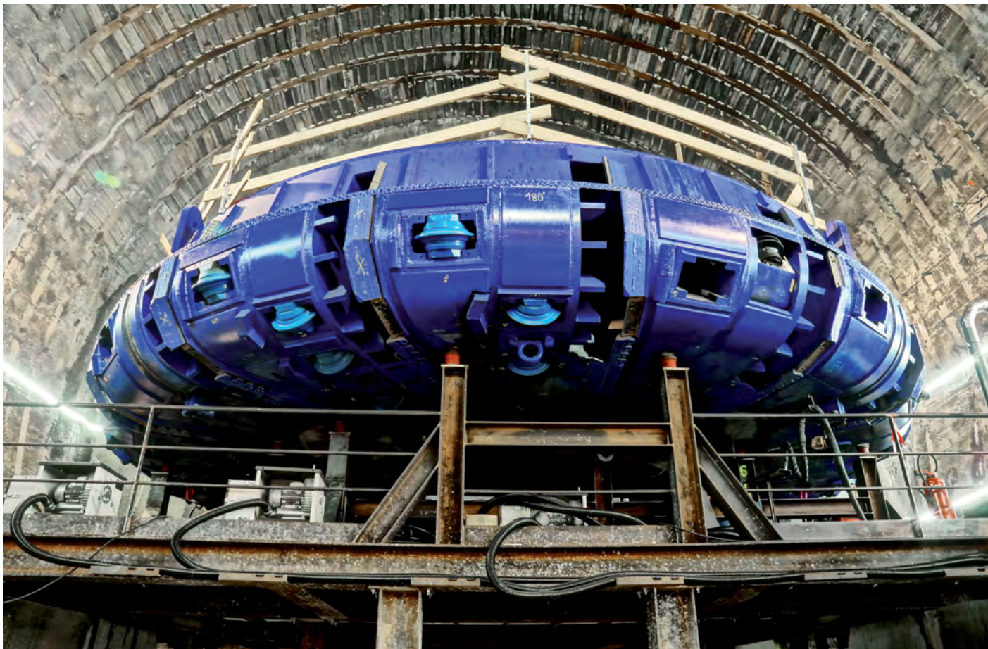
France, St. Martin La Porte - Turin-Lyon high speed railway
