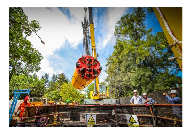
The Ghellas usually assemble the machine in-situ, so that it can better adapt to the characteristics of the ground and ensure an exemplary job.
