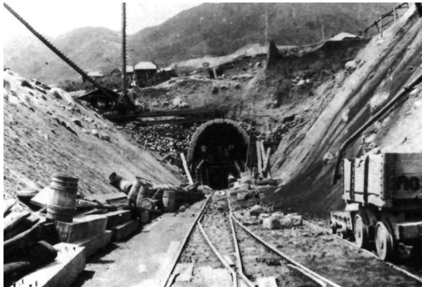
Beacon Hill Tunnel under construction, 1909, Hong Kong, China
