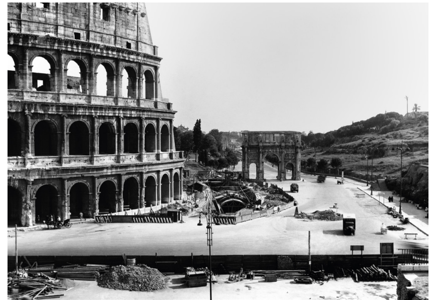
Colosseum metro tunnel, Rome, Italy
